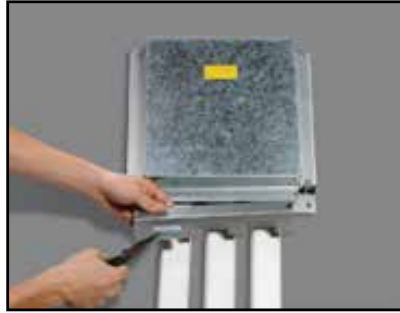
2-Peel off the pre-punched knock-outs at the side blank plate before laying the ductings
