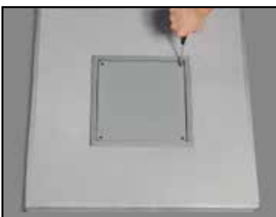
7.2- Mount the trap frame and trap cover.
